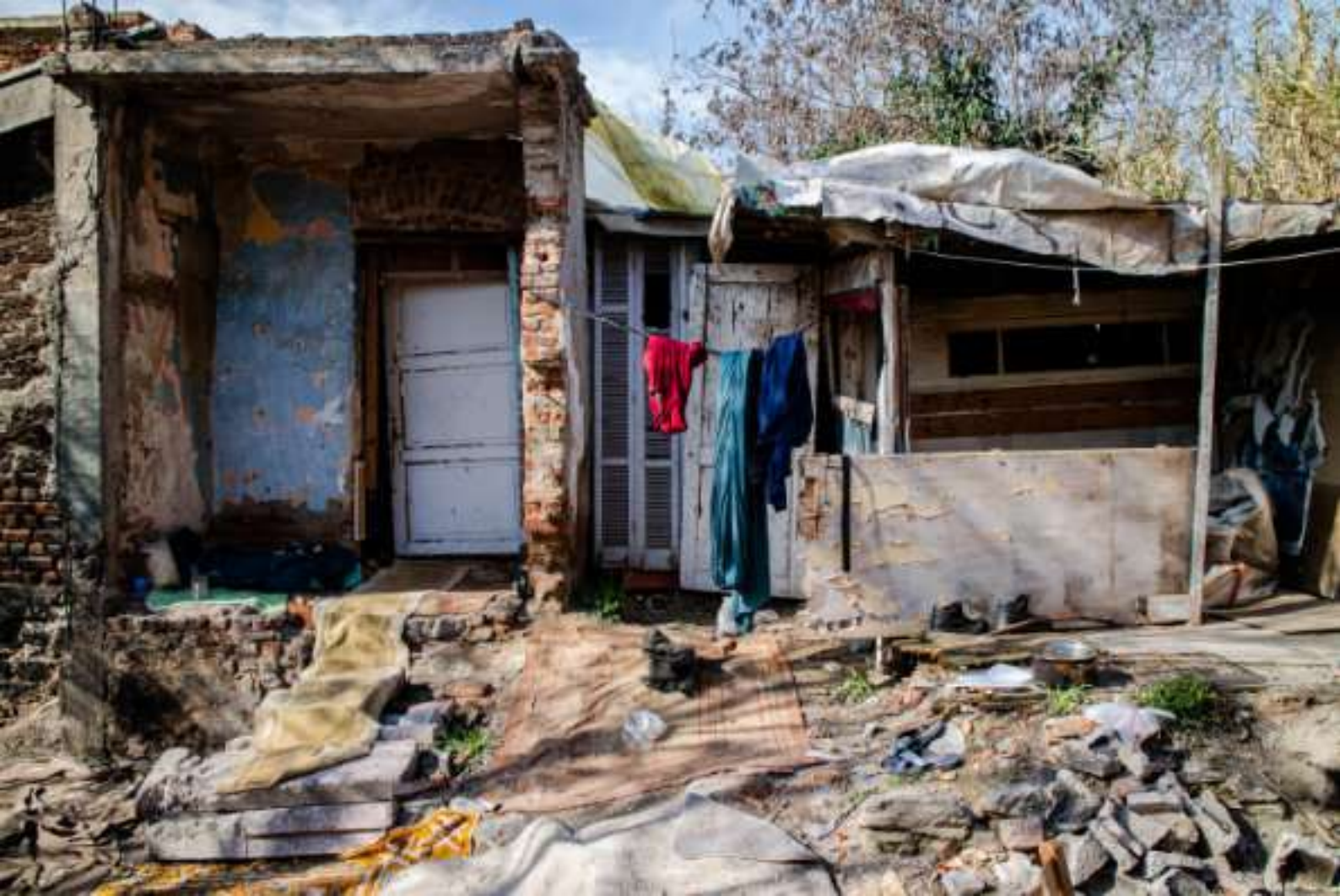
Abandoned building used as a squat Thessaloniki and surroundings Benji Herren 2021
