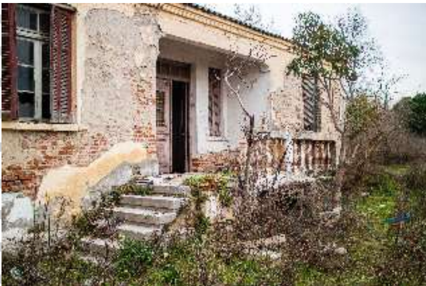
Abandoned building, Thessaloniki and surroundings Benj Herren 2021
